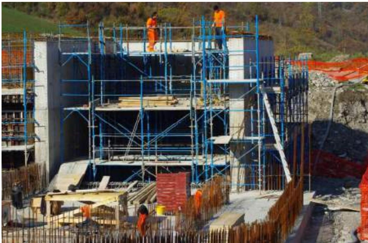
VASCA DISSABBIATRICE E DI MESSA IN CARICO – INCASTELLATURE PER ARMATURA SOLAIO
