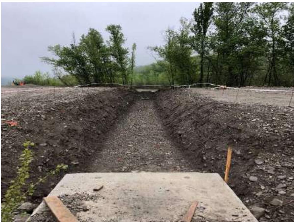
VASCA DI CARICO E DISSABBITORE – SCAVO POSA CANALE SCARICO DISSABBIATORE
